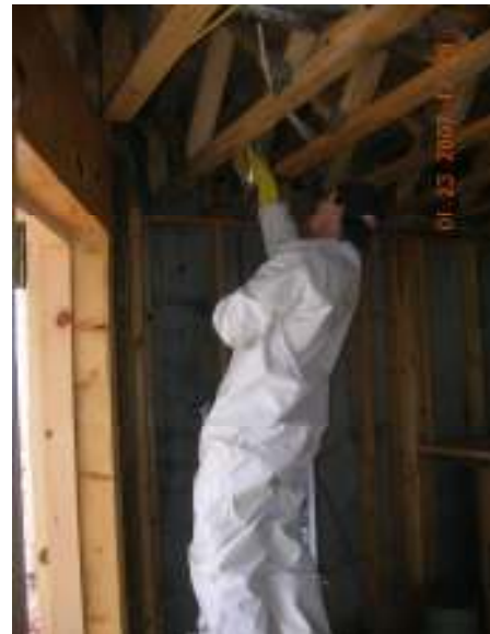
Fungal Contamination due to high air moisture
