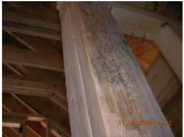
Fungal Contamination due to high air moisture
